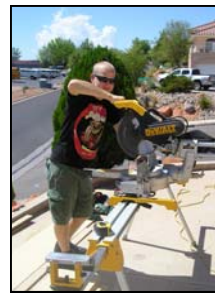
Richard S. Works with Jesse to install shelving..
